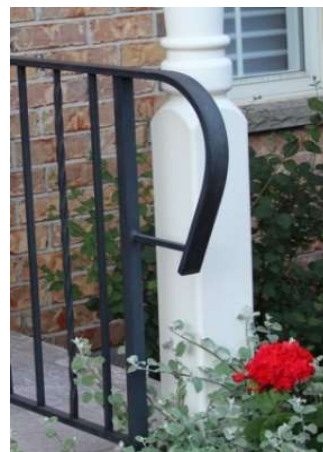
Railing on front porch of a one storey model
