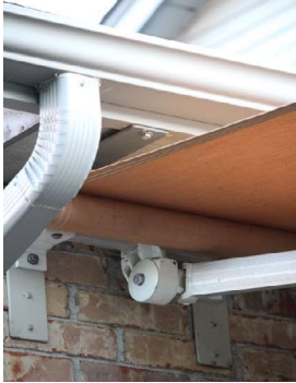
Proper fastening of awnings to the wall
