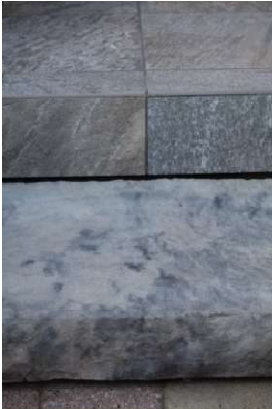
Landing/porch with approved exterior tile and new one piece flagstone step
